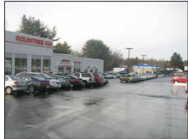
A properly cleared lot prevents slip/fall injuries.
